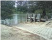
Concrete ramp - Lions Park Seymour
