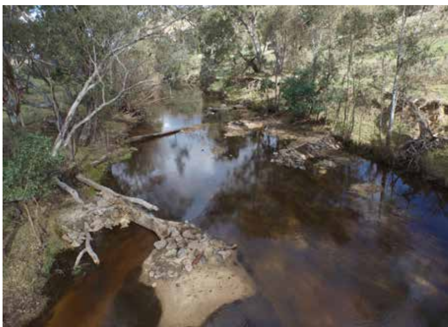
Figure 5: Instream habitat works – large wood and boulders placed to encourage depth in channel and sand deposition along bank.
