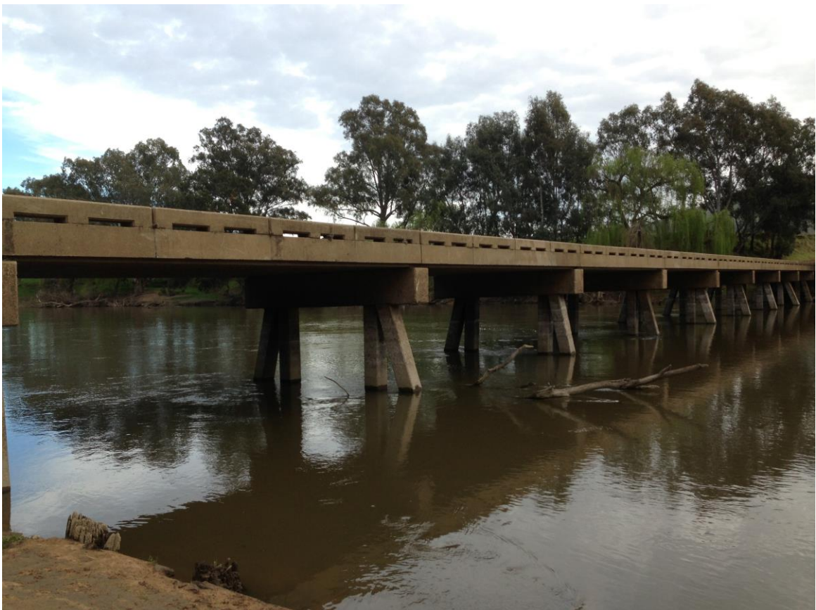
Figure 8 Mundarlo Bridge on the Murrumbidgee
