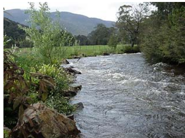
Site for bank stabilisation works - Stevenson River
