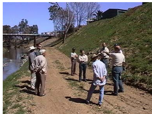
Inspecting Goulburn River bank stabilisation work Mooroopna
