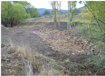
Rock chute constructed on Geoff Alford property April 2003
