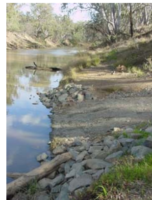
Reconstructed rock and stabilised rock filled launch ramp
