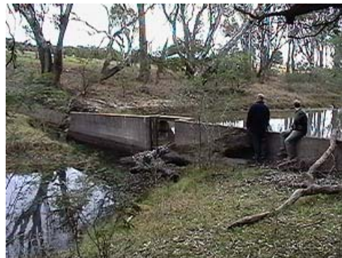
This redundant weir on Schiers Lagoon has been removed
