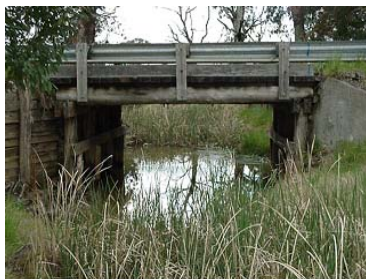
Location for bridge replacement - Prices Creek, Willowmavin
