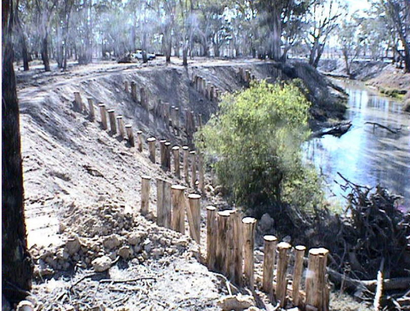
Photograph: Example of bank restoration works
