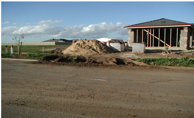
Building and construction sites continue to have a major impact on the degradation of stormwater quality
