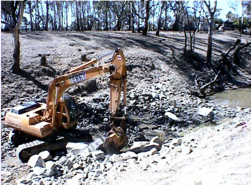
Photograph: Example of remodelling grade control structures
