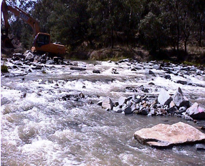
Photograph: Fish passage works, Goulburn River, Shepparton Weir
