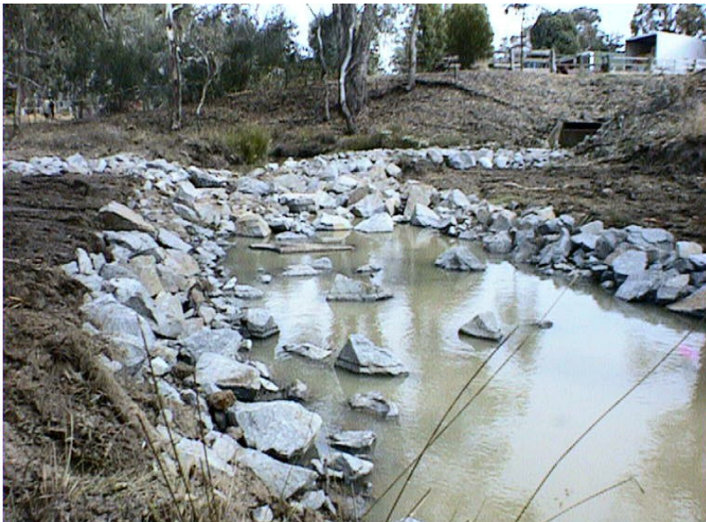
Photograph: Works on the Castle Creek
