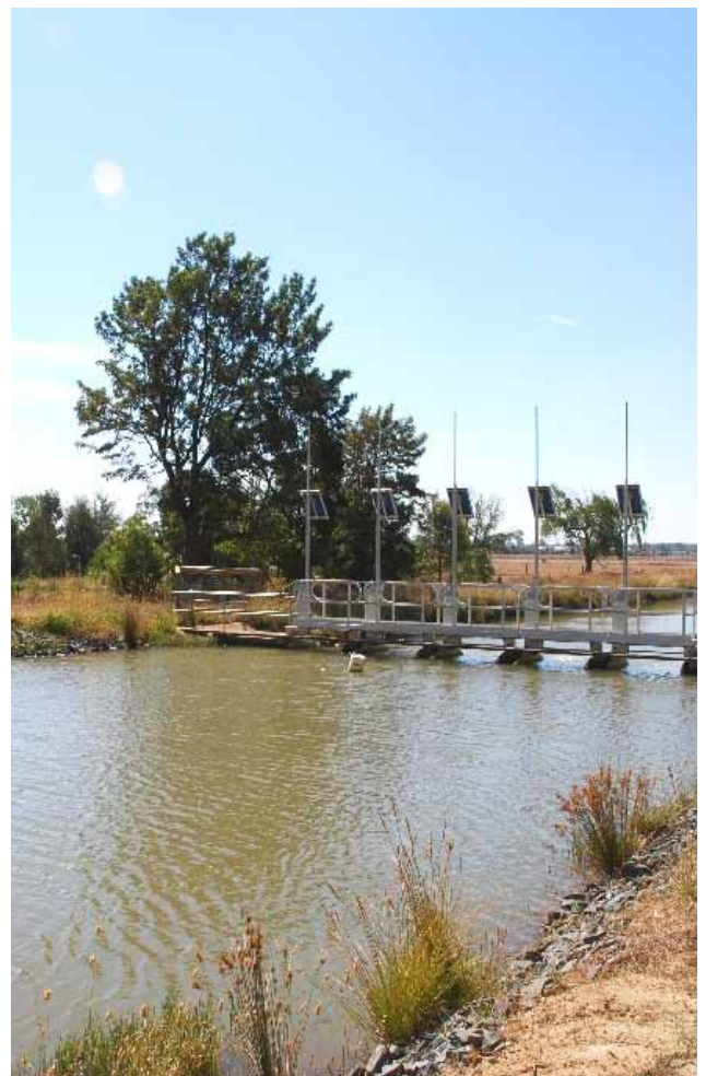
A modernised irrigation structure in the Shepparton Irrigation Region
