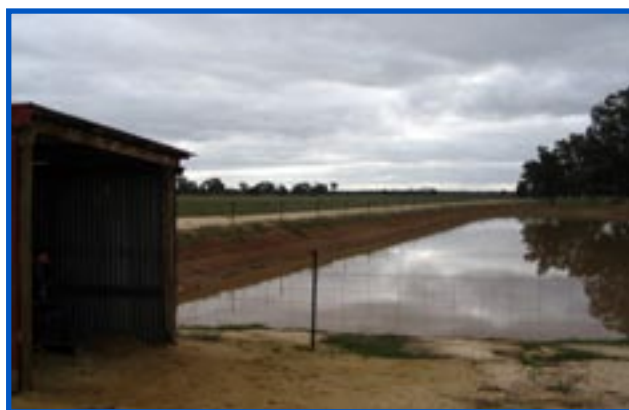
Reuse system installed with incentive scheme Automatic Irrigation Program
