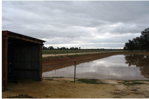
Re-use system installed with incentive scheme
