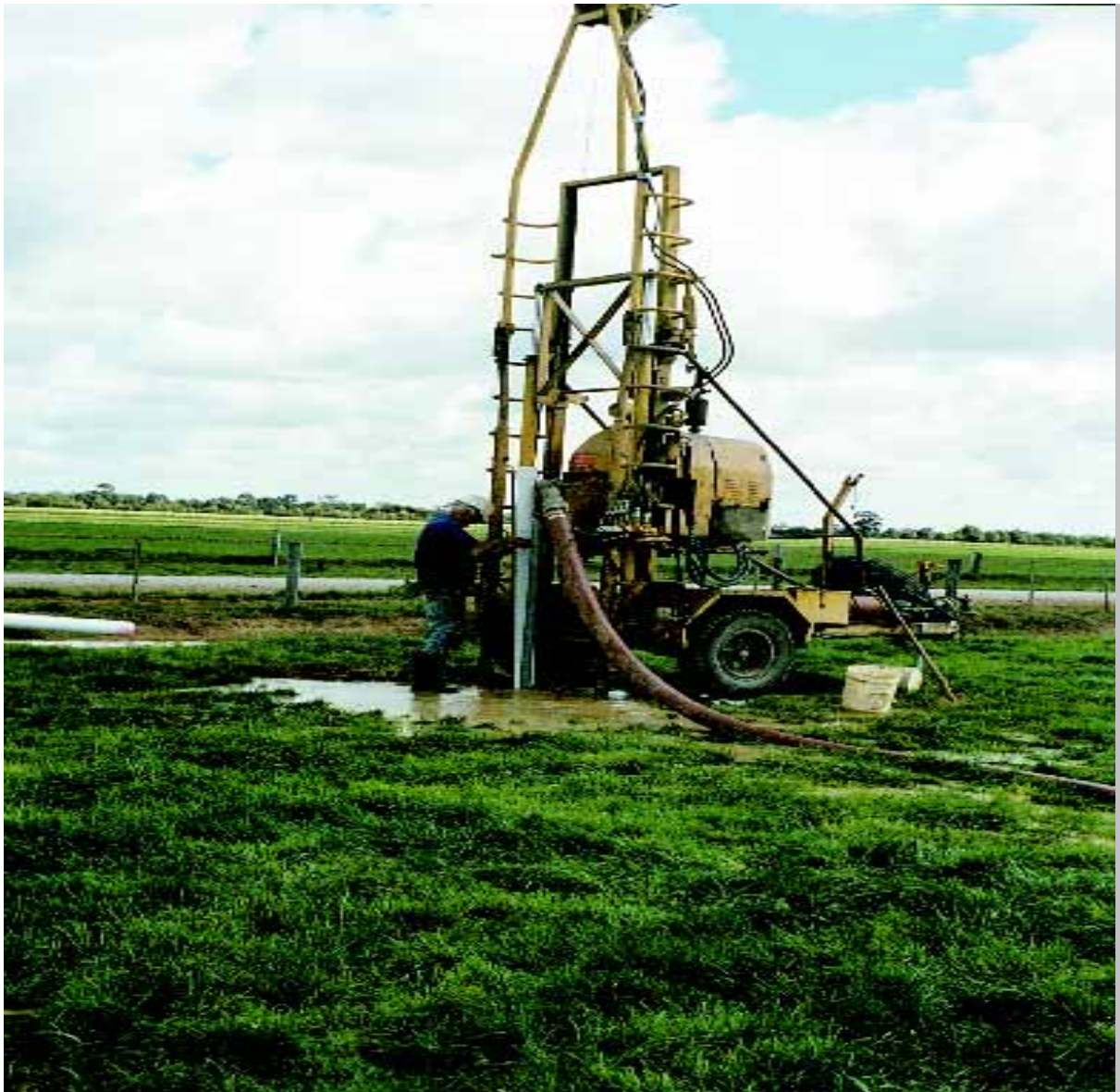
Figure 11 – Farm Exploratory Drilling
