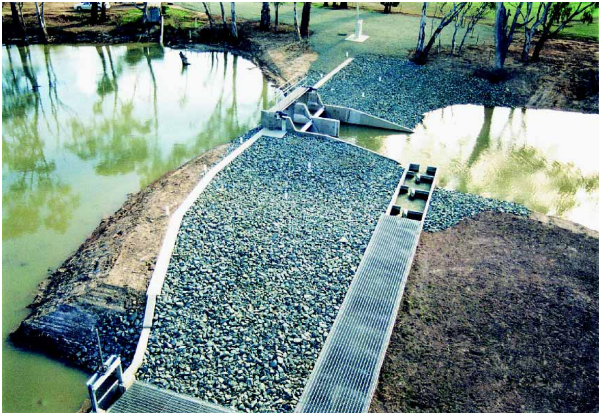
Figure 25 – Broken Creek Fish Ladder
