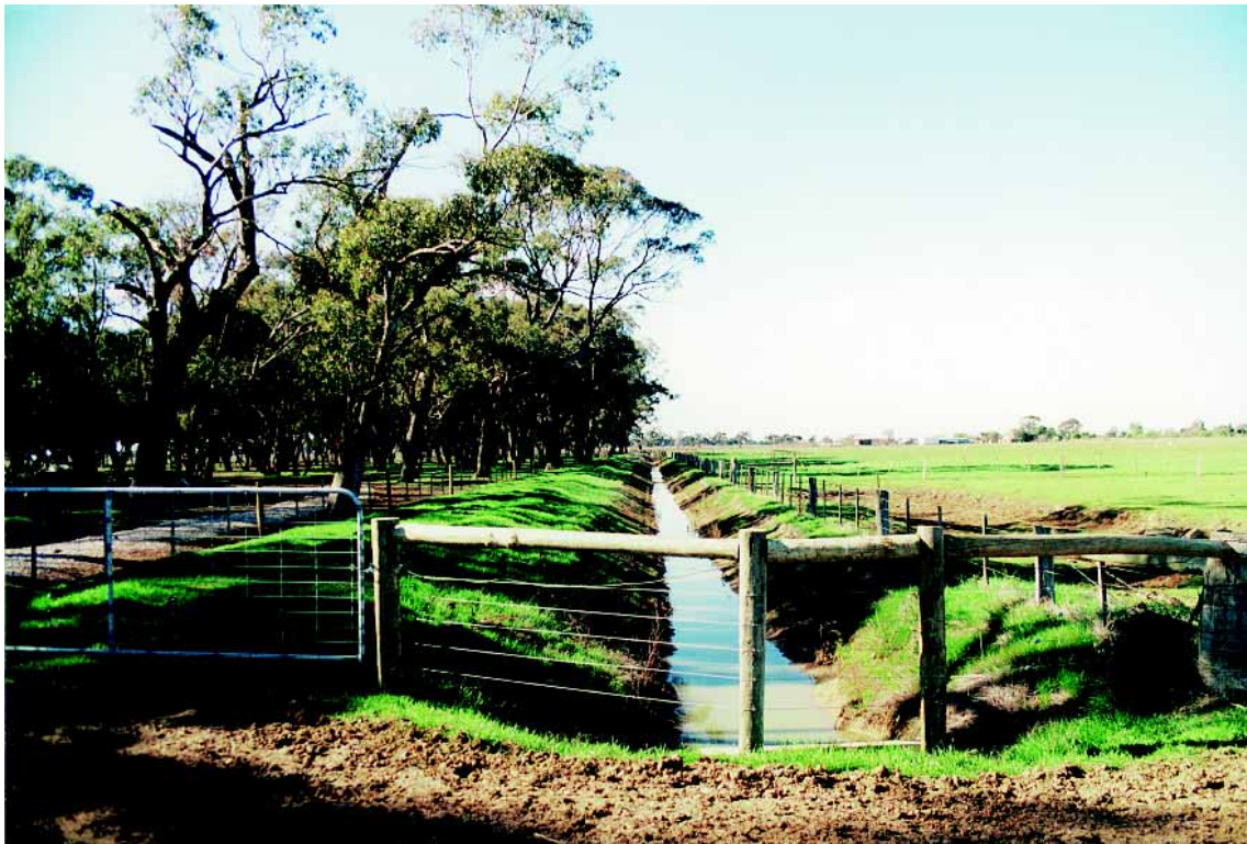
Figure 7 – Mosquito 23 Community Surface Management Scheme
