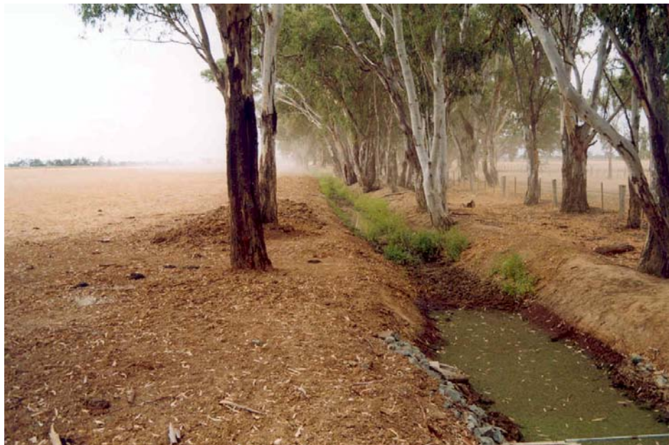
Figure 13 – Remodelled Surface Water Management System allowed trees to be saved Note that there is no maintenance track. This section will be sprayed for weeds by hand.
