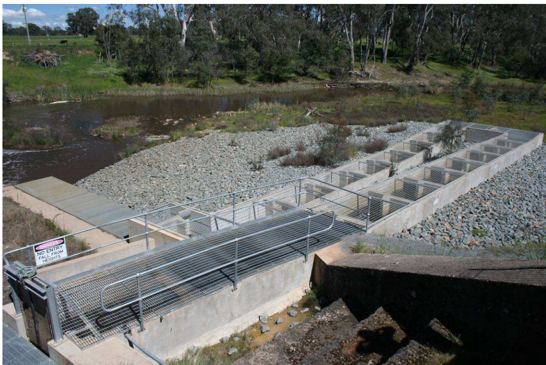
Figure 4. Vertical slot fishway on Casey's Weir. Photo: Rick Stoffels.
