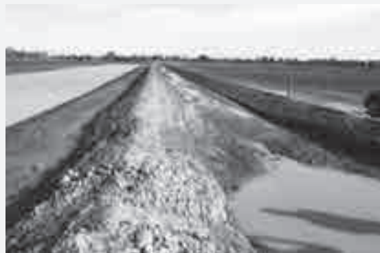
Channel constructed to deliver water from reuse system.
