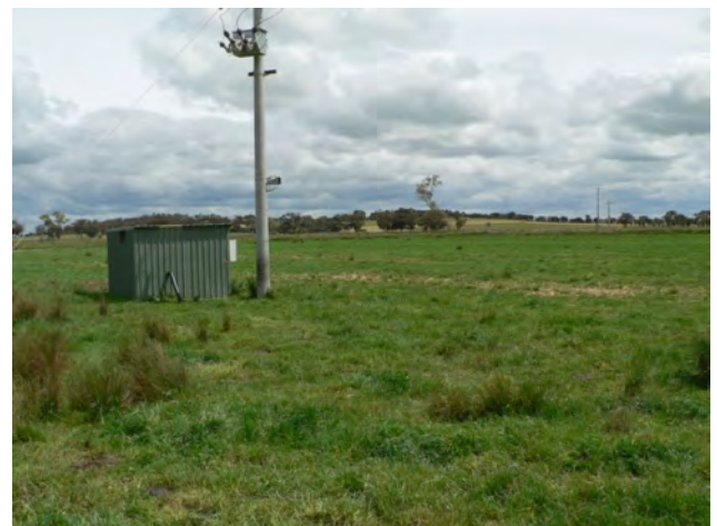
Groundwater pump shed with Mount Scobie in the background
