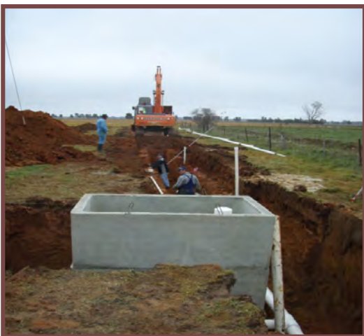
Picture: Header line and well-point installation
