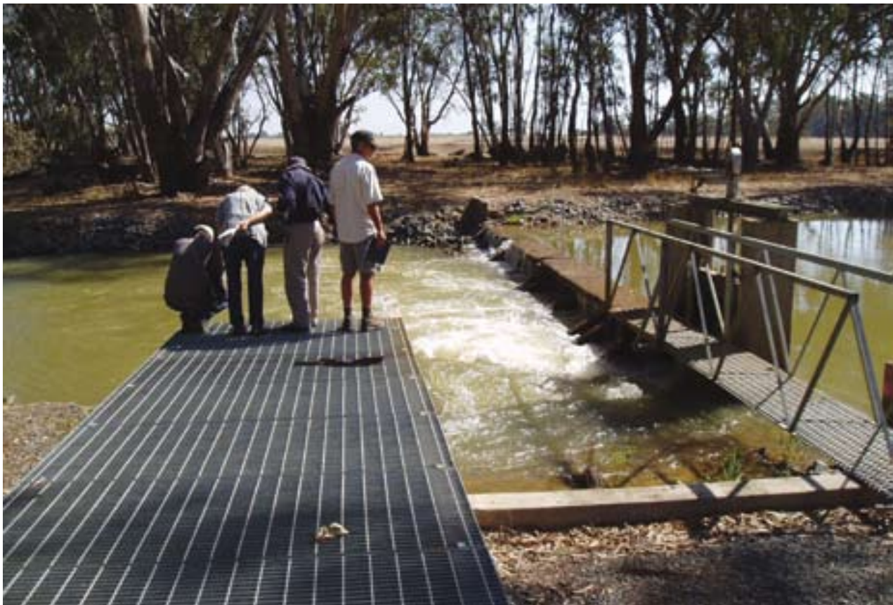
Flow through the Katandra Weir is monitored.
