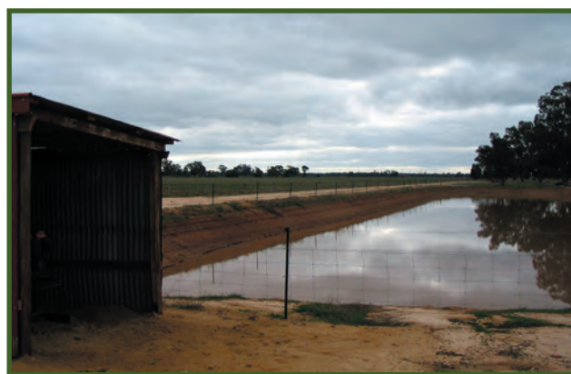
Re-use system installed with assistance from the drainage re-use project
